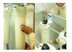
**Step 3**. Use a filter wrench (SW4 or similar) to carefully remove the sump from the filter housing
